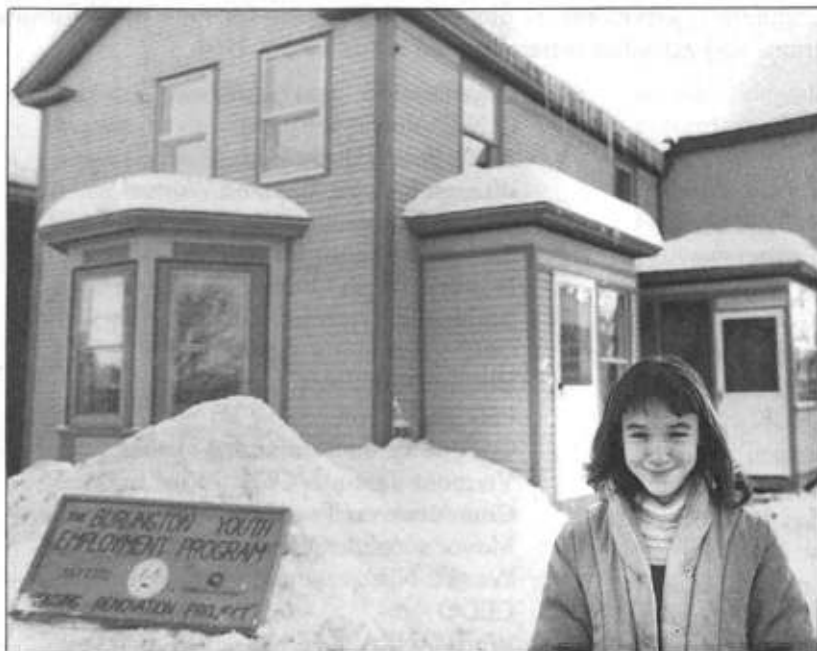
House renovated through Burlington Youth Employment Program.
